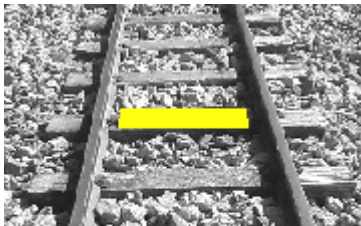
Yard limit track marker. See Rule 93.
